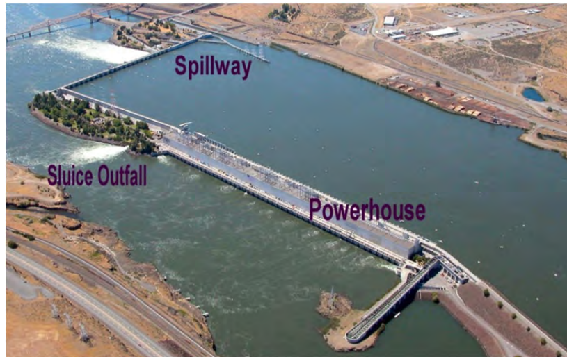
Figure 1.1. Aerial Photograph of The Dalles Dam
