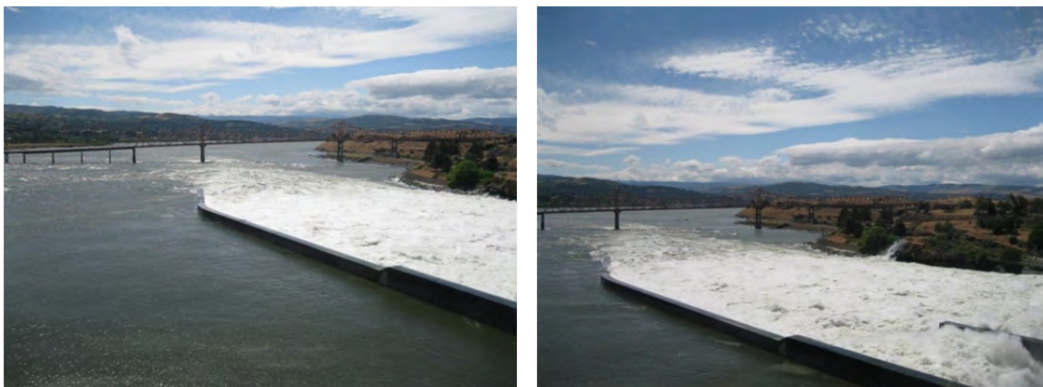
Figure 1.4. Photographs of The Dalles Dam Stilling Basin and the New Spill Wall (looking downstream)
