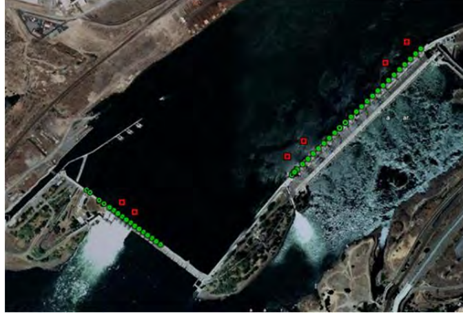
Figure 2.7. Location of Hydrophones on the Dam Face and in the Forebay of The Dalles Dam, 2010. The green and red symbols represent dam-face and clump mount hydrophones, respectively.
