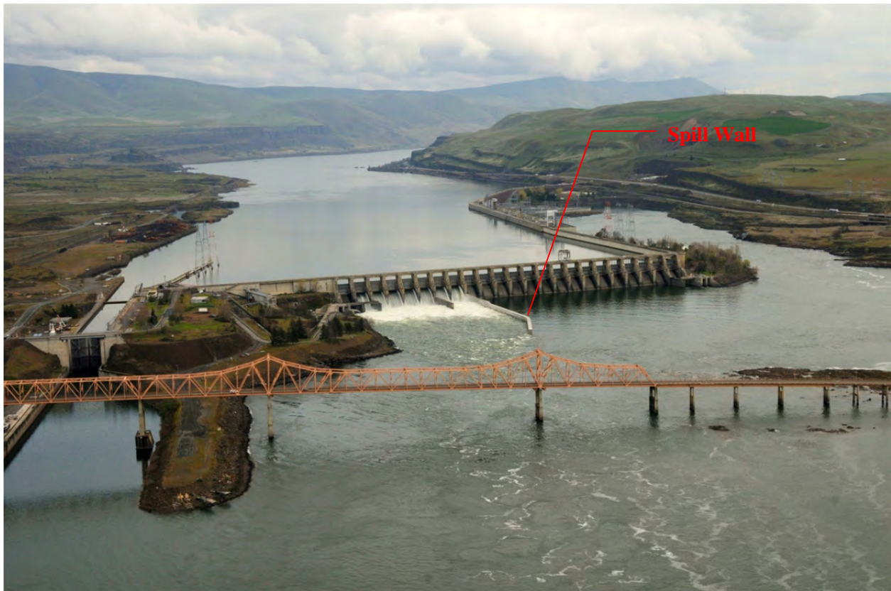
Figure 1.2. The Dalles Dam Spillway Showing the New Spill Wall at Bays 8/9
